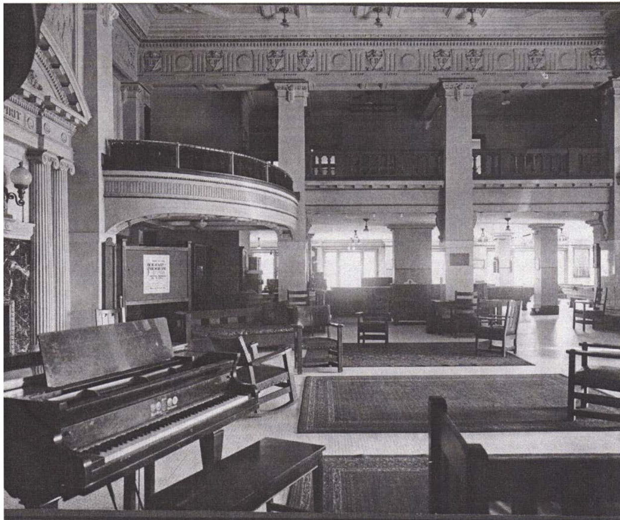
Figure 22. View of main lobby looking northeast, 1910. Courtesy of San Francisco YMCA.
